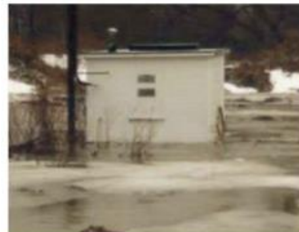
Historic Photo of Flooding Around Well House No. 2
