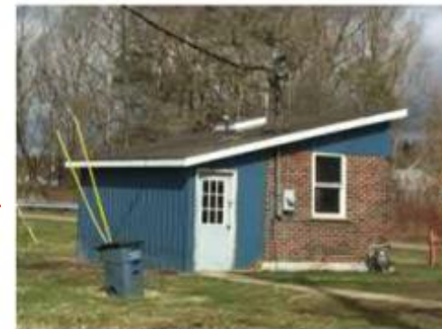
Well House No. 1
