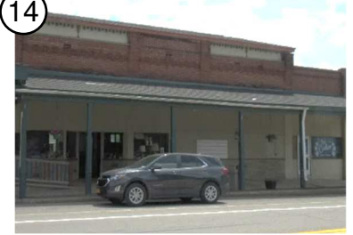
110 W. Main SBL:328.10-2-20 Old Hardware Shop Owner: Charles McDonnell
